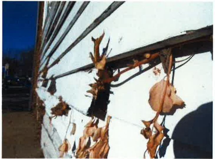
Encroachments behind the existing siding.
