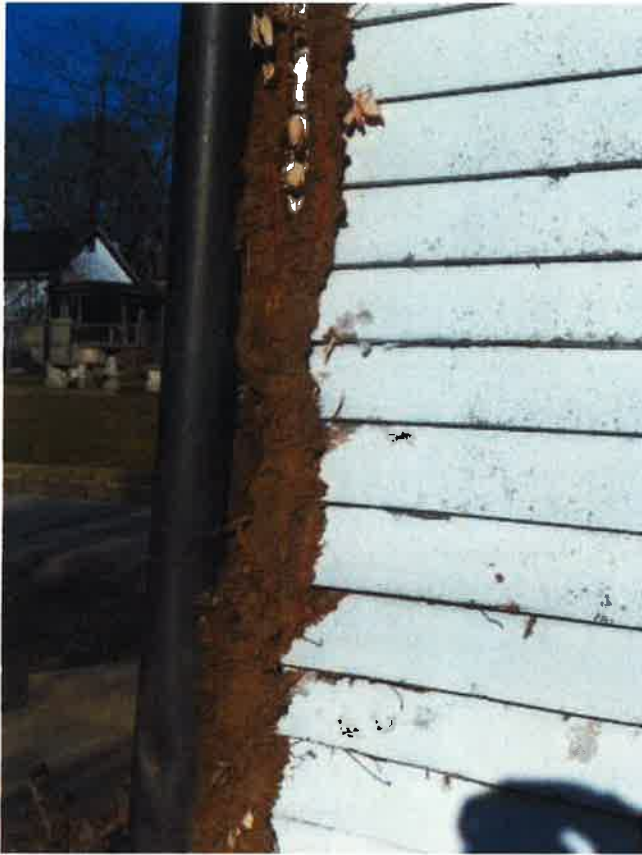
Remnants of vines that remain attached to the siding.
