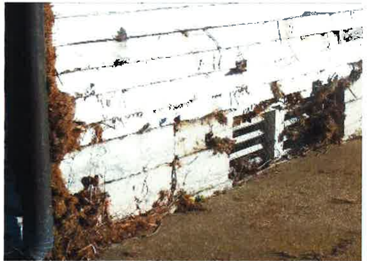
Additional encroachments around foundation and vents.
